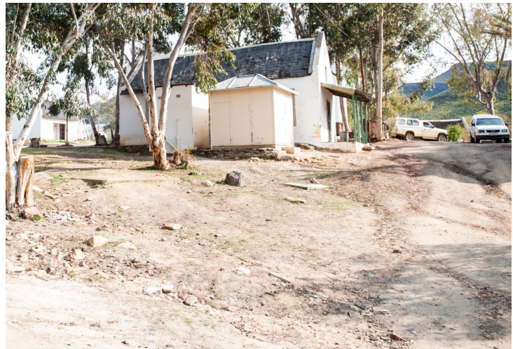
Fig. 7.49 Erosion next to post office (Franklin 2015)
