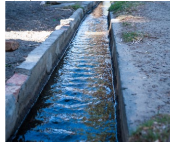
Fig. 6.37 Irrigation channel (Franklin 2015)
