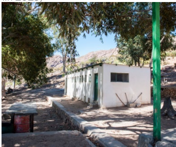
Fig. 6.32 New toilets on school yard (Franklin 2015)
