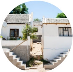
Steps at residential home
