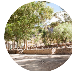
2. Retaining rock walls
