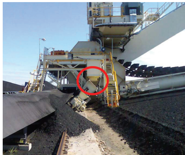
Figure 2—Failure of the bogie on a portal reclaimer
