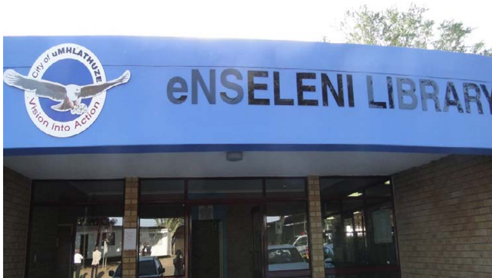
Figure 10: eNseleni Library Entrance, 2011
