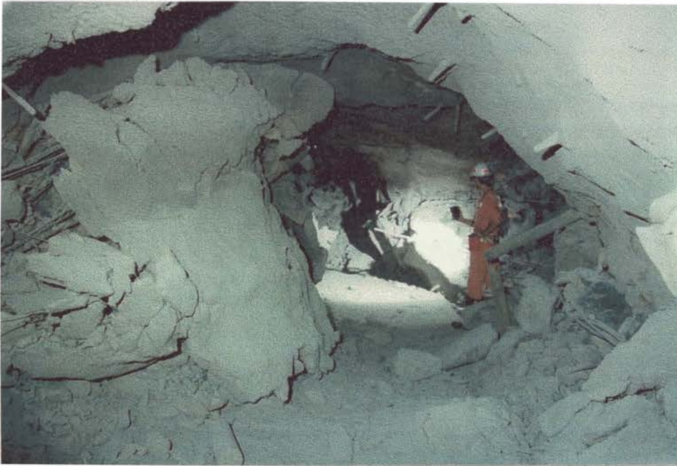
P.A. 10. DS5 on Damage Scale. Tunnel 109 collapse on 583 metre level in pillar in Tuffitic Kimberlite Breccia. (RMR 52)
