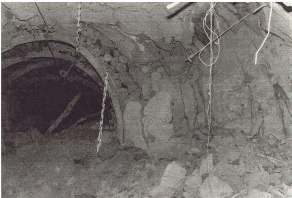
P.A.9. DS5 on Damage Scale. Collapse of steel arches, induced fracturing and dilation on pristine and induced fracturing around tunnel 120 on 568 metre level in Tuffisitic Kimberlite Breccia (RMR 48) in stressed pillar.
