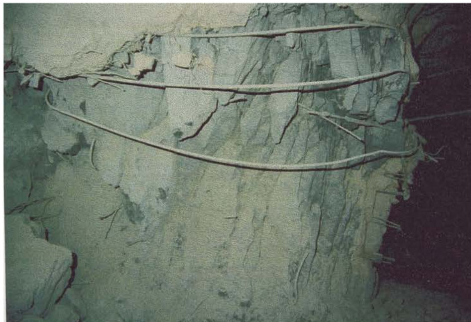
P.A. 13. Induced fracturing in Hypabyssal Kimberlite after drawbell development and undercutting (MRMR 34).
