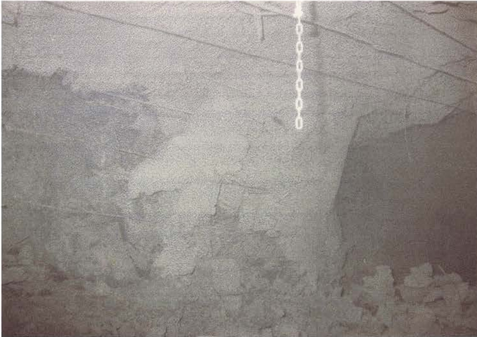
P.A.6. DS3 on Damage Scale. Damage to support and underlying rock on 630 metre level after undercut has passed overhead.
