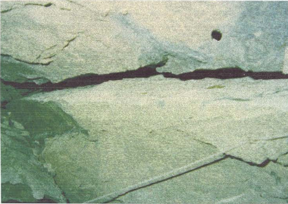
P.7.1. Dilation (20mm) on joint in TKB prior to caving
