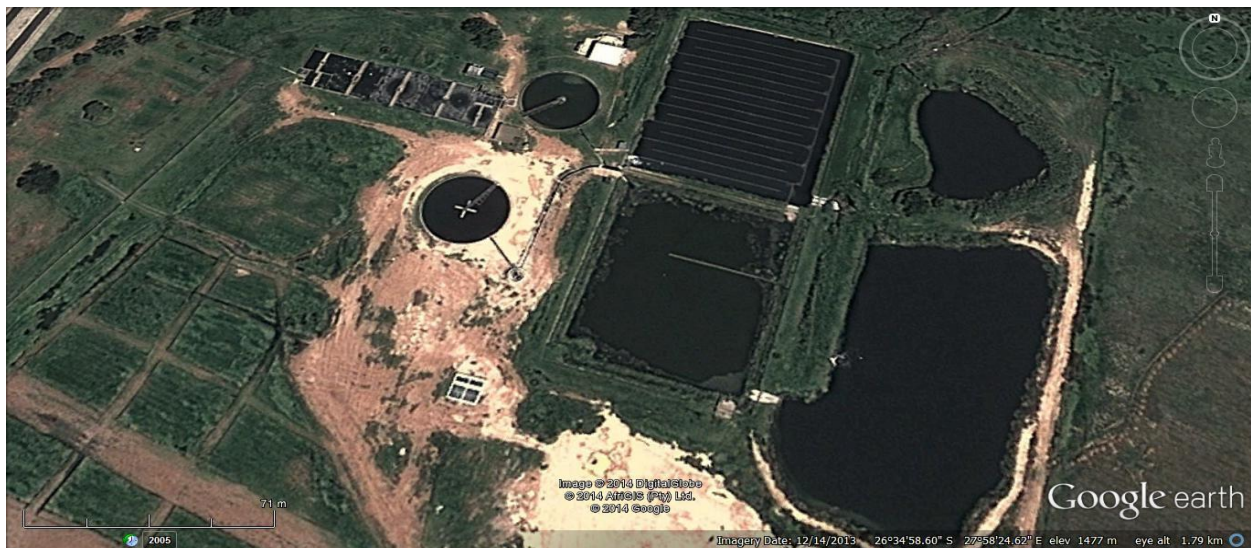
Figure 3.13: Satellite image of the Meyerton WWTP4
