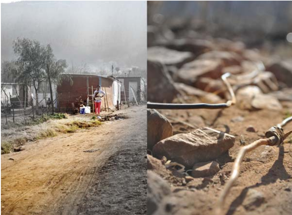
Figure 5.39: Visual documentation of illegal water and electrical connections (Maritz 2011)
