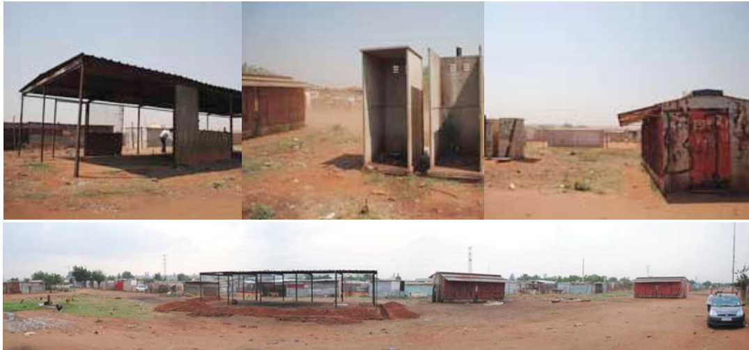
Figure 5.24: Photographic documentation of existing conditions (Bennett et al 2010)
