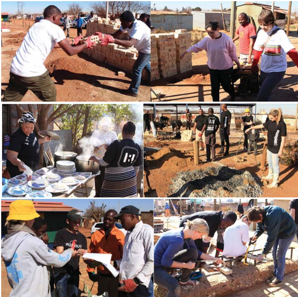
Figure 5.99: Construction activity on the site (1to1 2014)
