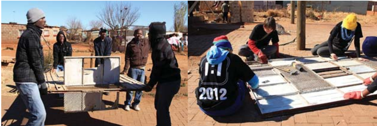
Figure 5.98: Existing steel windows held in storage by the SPCDF that were used to enclose the hall (Horzook 2012)
