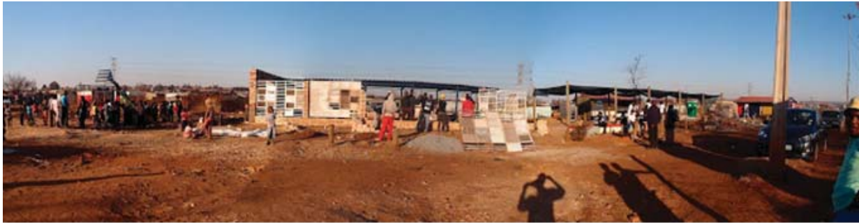
Figure 5.100: Construction in progress (Bennett 2012)
