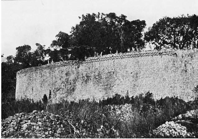
Figure 124 Great Zimbabwe, view of southeast wall of Great Enclosure. The stelae are arranged above a chevron pattern in the top part of the wall. (Randall Maclver, 1906) https://commons.wikimedia.org/wiki/File:Exterior_of_great_enclosure,G.Zimbabwe.JPG
