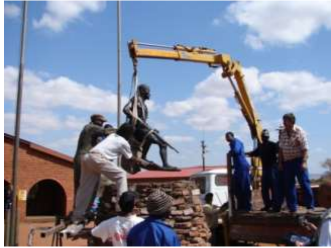
King now in bronze still in 14 pieces welded together with TIG Statue placed on pedestal and unveiled
