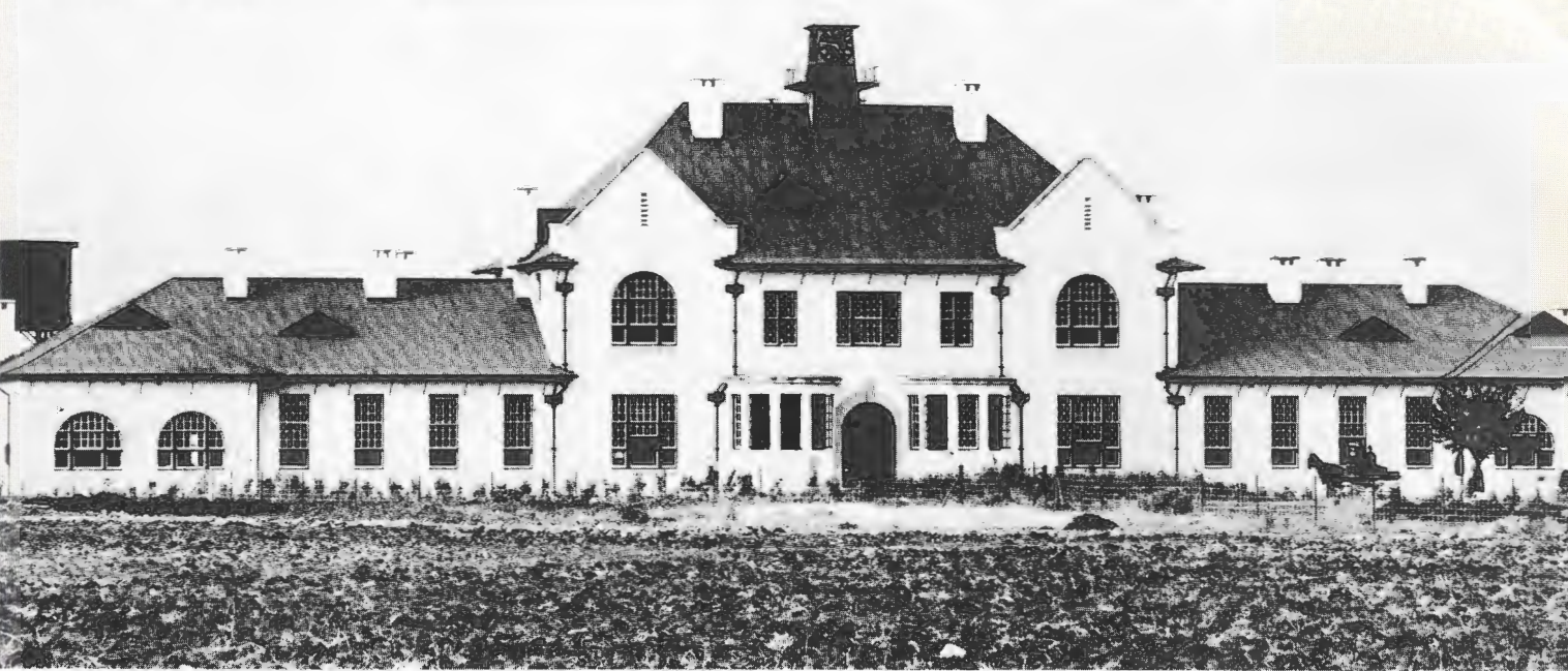
The main building of the Onderstepoort Bacteriological Institute (later Veterinary Research Institute) shortly after it was ready for use in 1908 but before the gardens and grounds were fully laid out.
