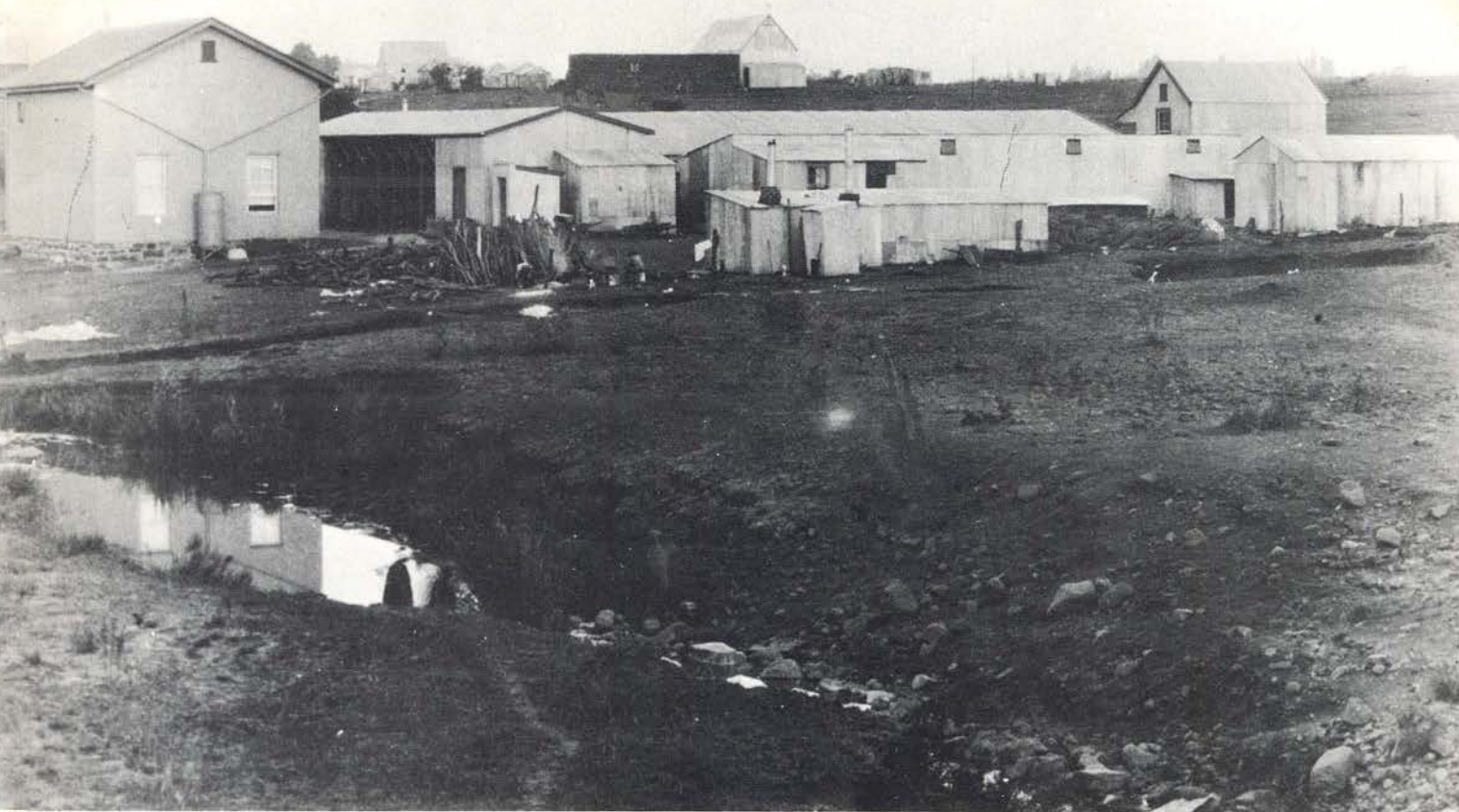
Daspoort Disinfection Station , built of wood and corrugated-iron and standing on boggy ground, which became in July 1898 the Z.A.R. Government Bacteriological Laboratory directed by Arnold Theiler.
