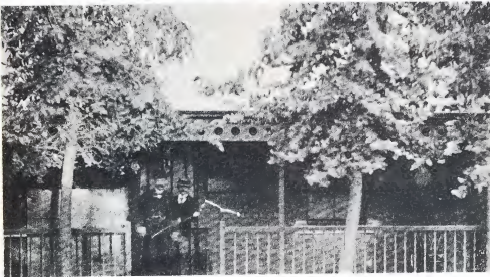
Brick and Corrugated-Iron House rented by the Theilers in van Wielligh Street, Johannesburg from 1893 to 1895. His plate may be seen to the right of the front door.
