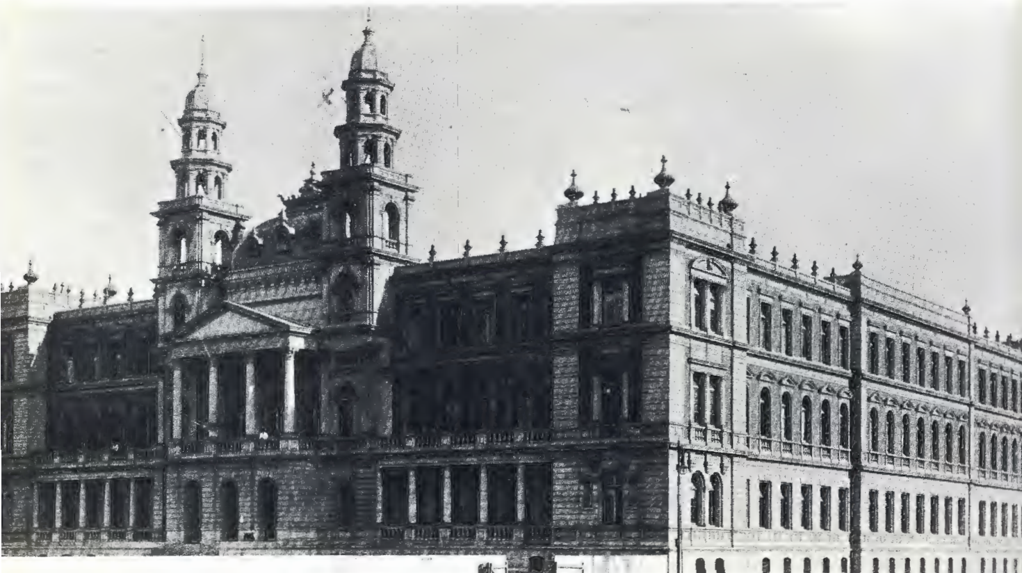
The Palace of Justice, Church Square, Pretoria in similar Renaissance style and completed some time after Theiler's arrival in the capital of the South African Republic.
