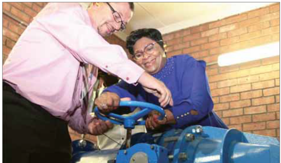
Figure 1: Jacques van Delft, Bloemwater electrical technician, helps Nomvula Mokonyane, Minister of Water and Sanitation, to open the water supply valve at the launch to get the turbines running
