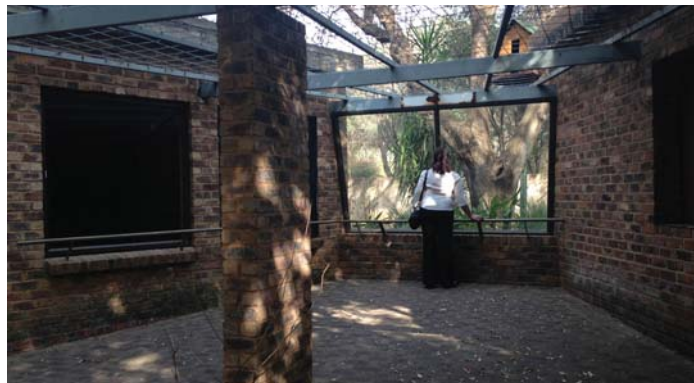
V_9. Existing primate cages on site (Author 2014).
