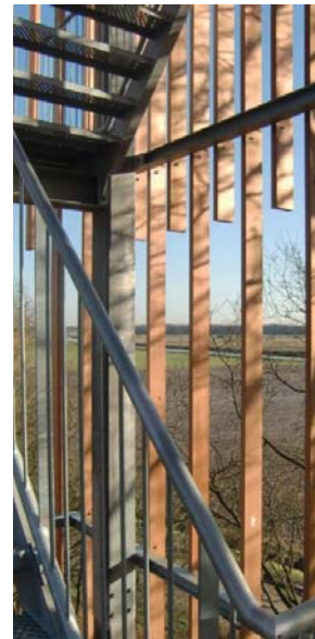
V_47. Viewingtower at Vecht Riverbank / Ateliereen Architecten (Archdaily 2012)
