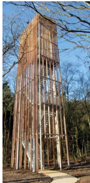
V_46. Viewingtower at Vecht Riverbank / Ateliereen Architecten (Archdaily 2012)
