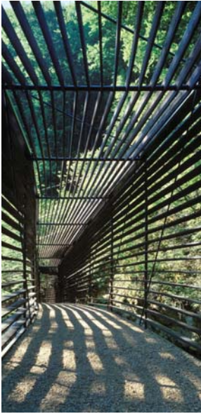
V_29. Footbridge Crossing L'Areuse (Architizer 2014).
