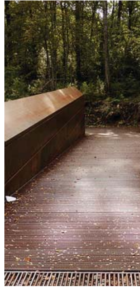
V_31. Re-bar footpath, RCR Architectes (Landezine 2014).
