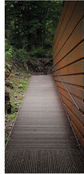
V_33. Re-bar walkway, Tussols basil sport- park, RCR Architects (Landezine 2014).
