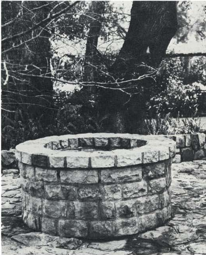
1. At the end of the Garden closest to Adderley Street, between the South African Library and the aviary, may be found a very old well, dated to 1842. Constructed of imported red brick, it has a depth of 2,7 m and a diameter of 1,12 m. At regular intervals down the shaft there is a wooden ring, on top of which rests a layer of shale through which the water filters into the well. The bottom of the well rests on white clay. Looking down into the well it is possible to see a small section of the original slate covering jutting out over the top of the red brick. The low sandstone wall and paving around the well were completed in 1980.
