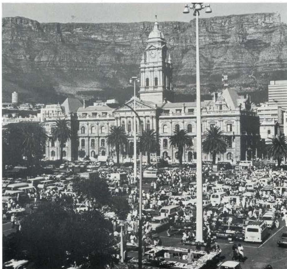
2. The Grand Parade: an area for which development guidelines have already been prepared.
