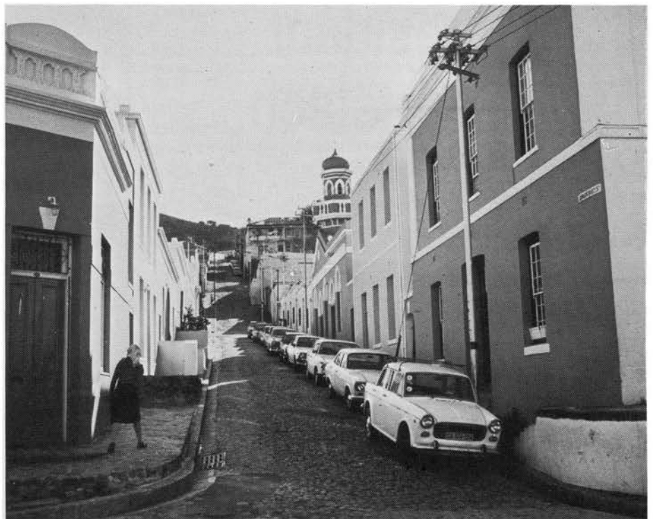
Chiappini Street, in the Malay Quarter: sensitive restoration.
