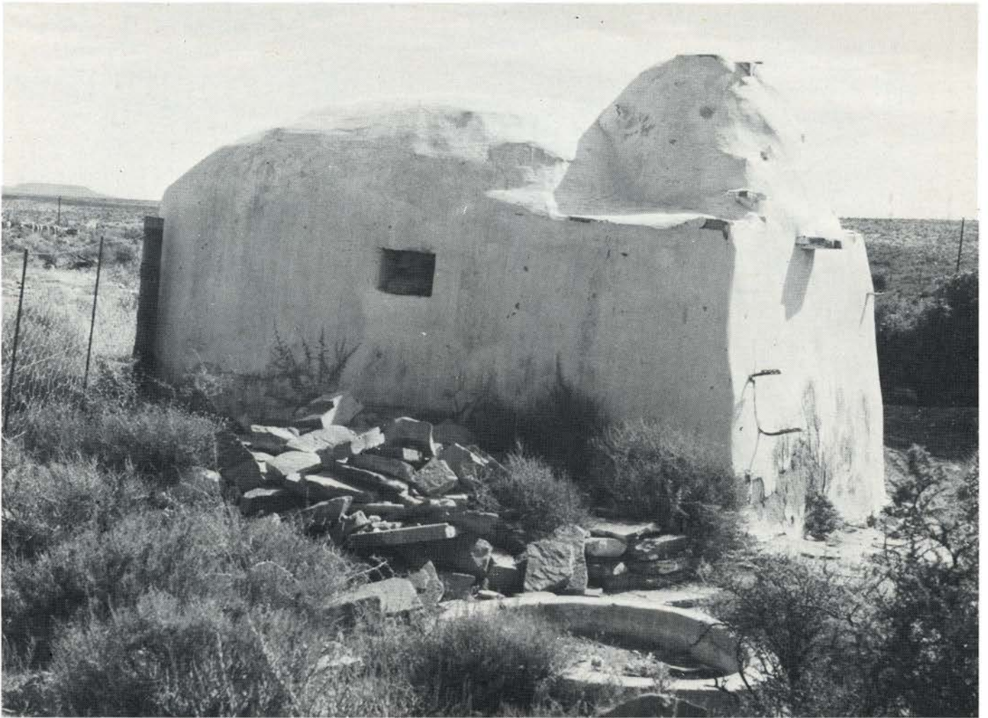
Fig. 3: Soap House — showing corbelled domed chimney stack, De Puts, Loxton
