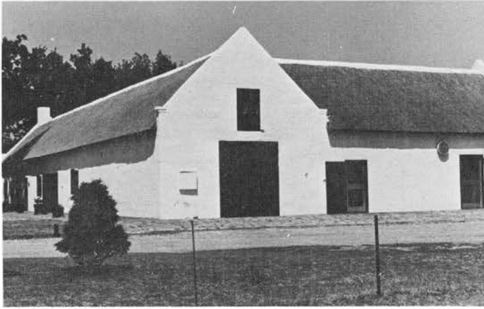
The north-east gable which was re-built to define the early rectangular formed building. The foot of the "L" shape extending to the right of the gable was a later addition.
