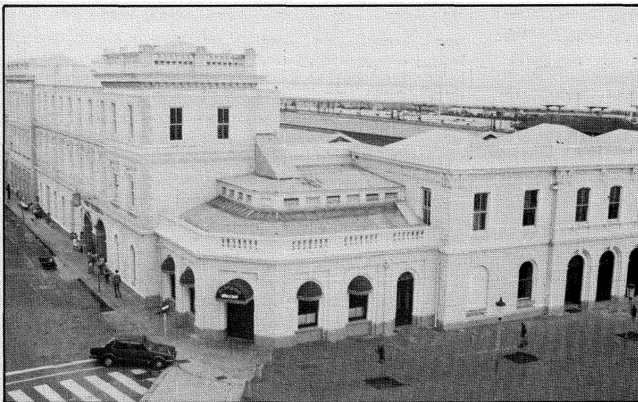
Port Elizabeth renovated station building — August 1985 Two-storey Georgian style building is the original station (1875). The remaining Victorian style buildings were added during the 1890s. Photograph taken from the elevated freeway. Algoa Bay in the background.
