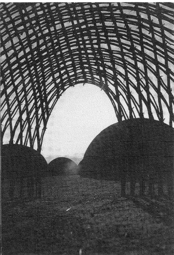
Reconstruction of Royal Residence, Ondini.
