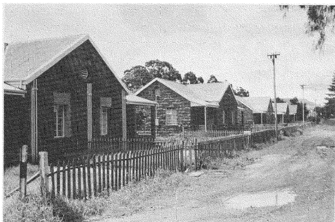
NZASM cottages at Volksrust Station. (Photo: the author)
