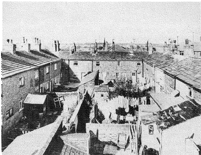
Courtyard 1975 before improvements showing outside toilets and wash-houses.
