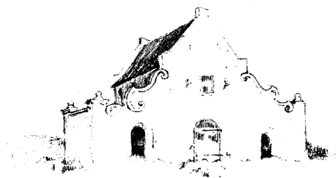
Pencil drawing of the devocote at Meerlust. This does not show the deterioration evident in a photograph by Arthur Elliott taken about 15 years later. (William Fehr Collection)
