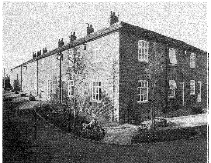
Holland Place showing new road parking bays, planting, improved dwellings.
