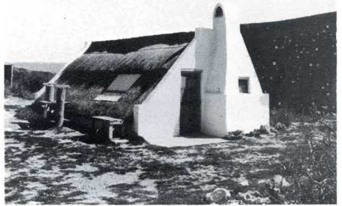
Fig. 10 Kapstylhuis with low side walls and gable hearth, Puntjie. Photo: James Walton
