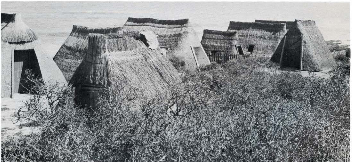
Fig. 2. Kapstylhuise , Puntjie. Dwellings sited at right-angles to the shore. Cooking-sheds, on the right, built parallel to the shore. (Photo: James Walton)
