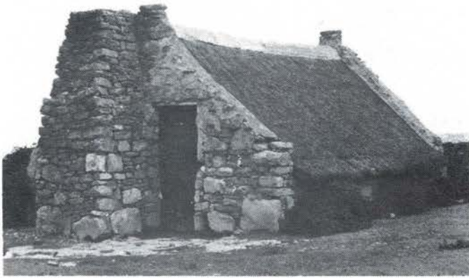
Fig. 9 Kapstylhuis with low rubble side walls and gable hearth, Vermaaklikheid. Photo: James Walton
