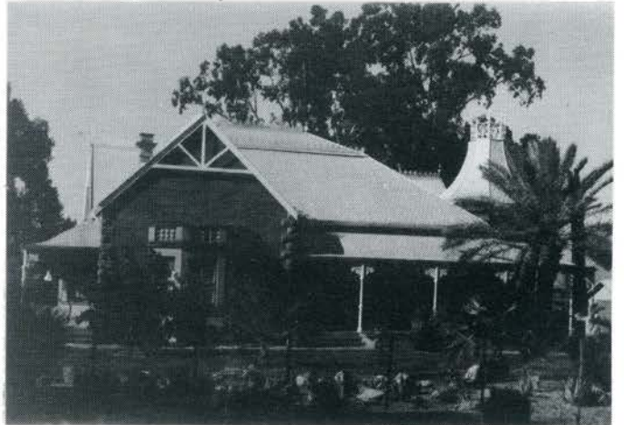
Front elevation of Schoeman's House
