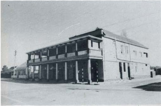
The Criterion Hotel. A new balcony and other alterations were added to the original building.
