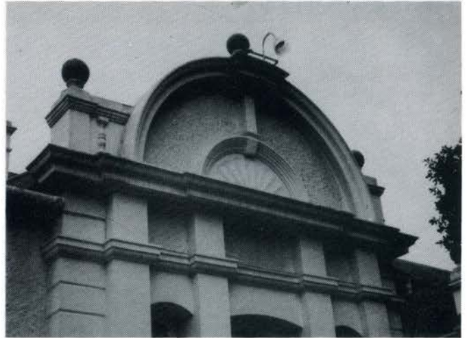
Detail of Gable
