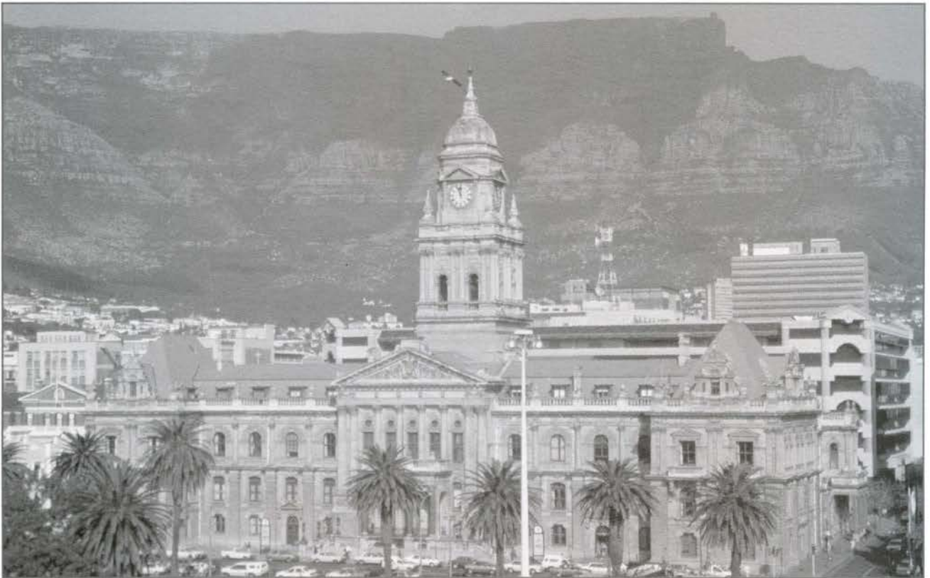
Cape Town City Hall – undergoing restoration by Gordon Verhoef & Krause
