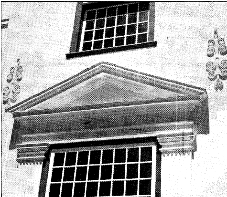
Fig. 11 Ornamental wall-anchors over the front entrance to Groot Constantia
