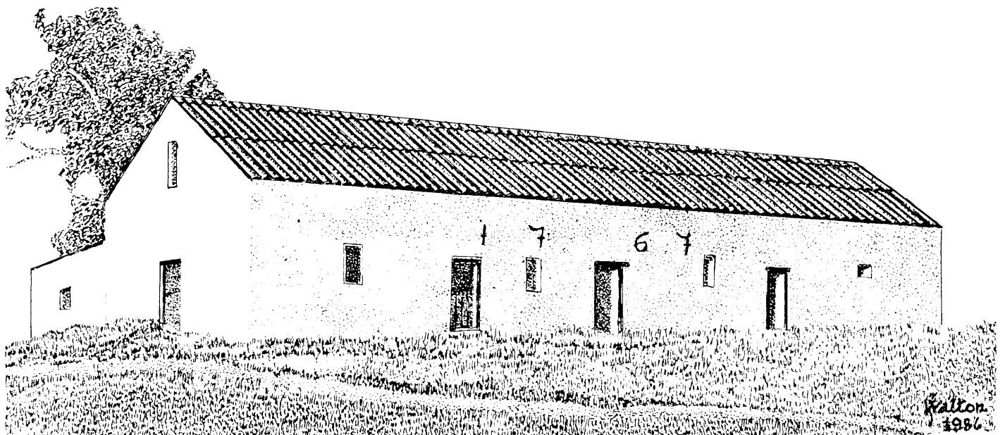
Fig. 1 A building with dated wall-anchors — Phesantekraal
