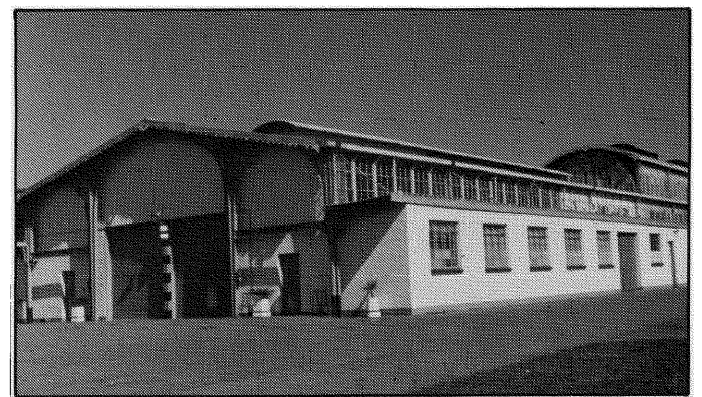
The steel and glass roof of the insular platform of the old Park Station, now at Esselen Park. The brick walls were added after the structure was re-erected at its present site. (Photo: the author)
