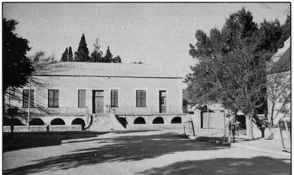
i) Before restoration
