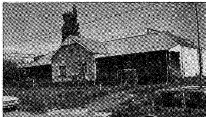
Double cottage of the larger type, Krugersdorp Station (Photo: the author)
