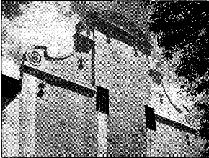
Fig. 10 The east gable of Groot Constantia, showing the present wall-anchors. Similar wall-anchors are now visible on the west gable
