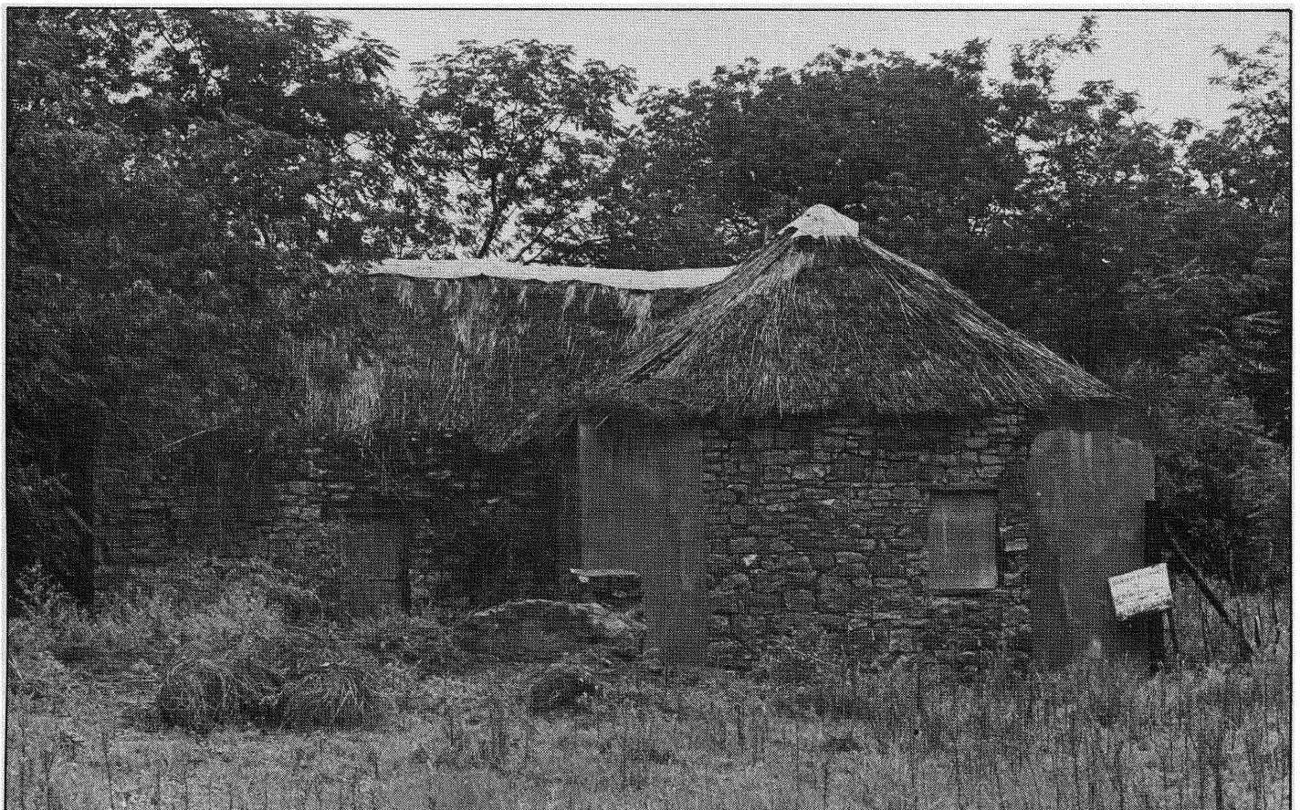
House from the south, prior to restoration.
