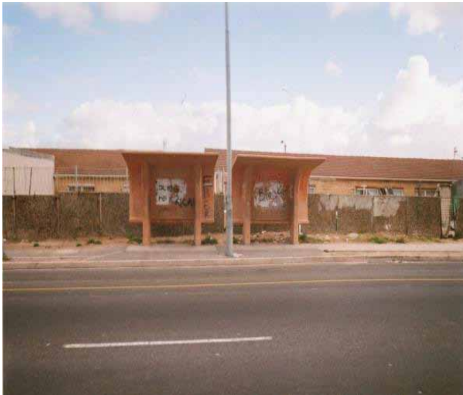
Figure 2 A view of a bus stop.
