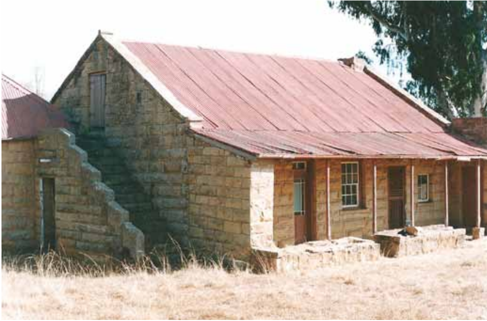
Figure 5 Sandstone masonry of Schoongezicht, 1883, replete with external staircase to the attic (source: Du Preez, 2012).
