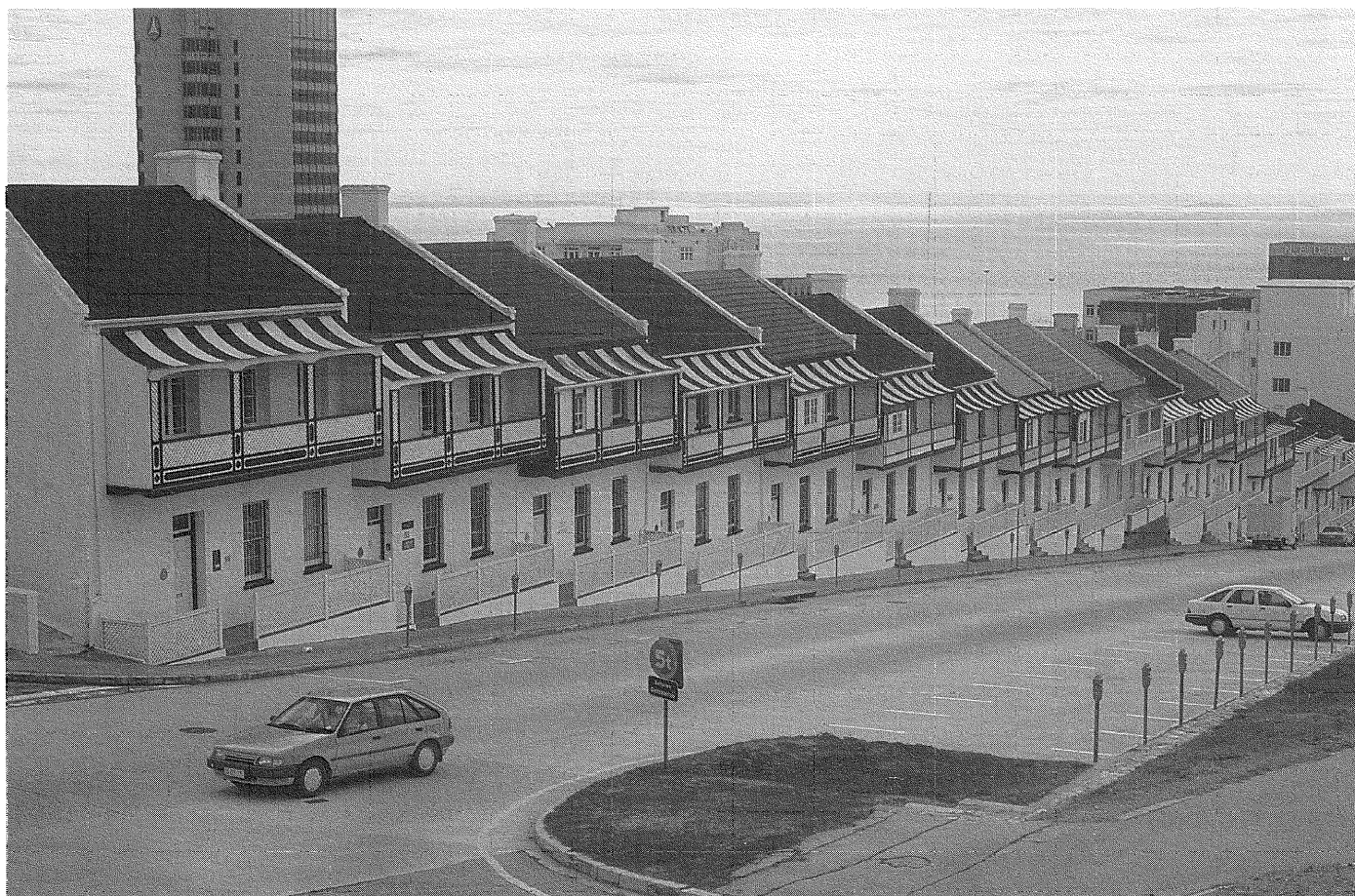
Donkin Street houses in Port Elizabeth restored by Nick Woolff serve as office accommodation
