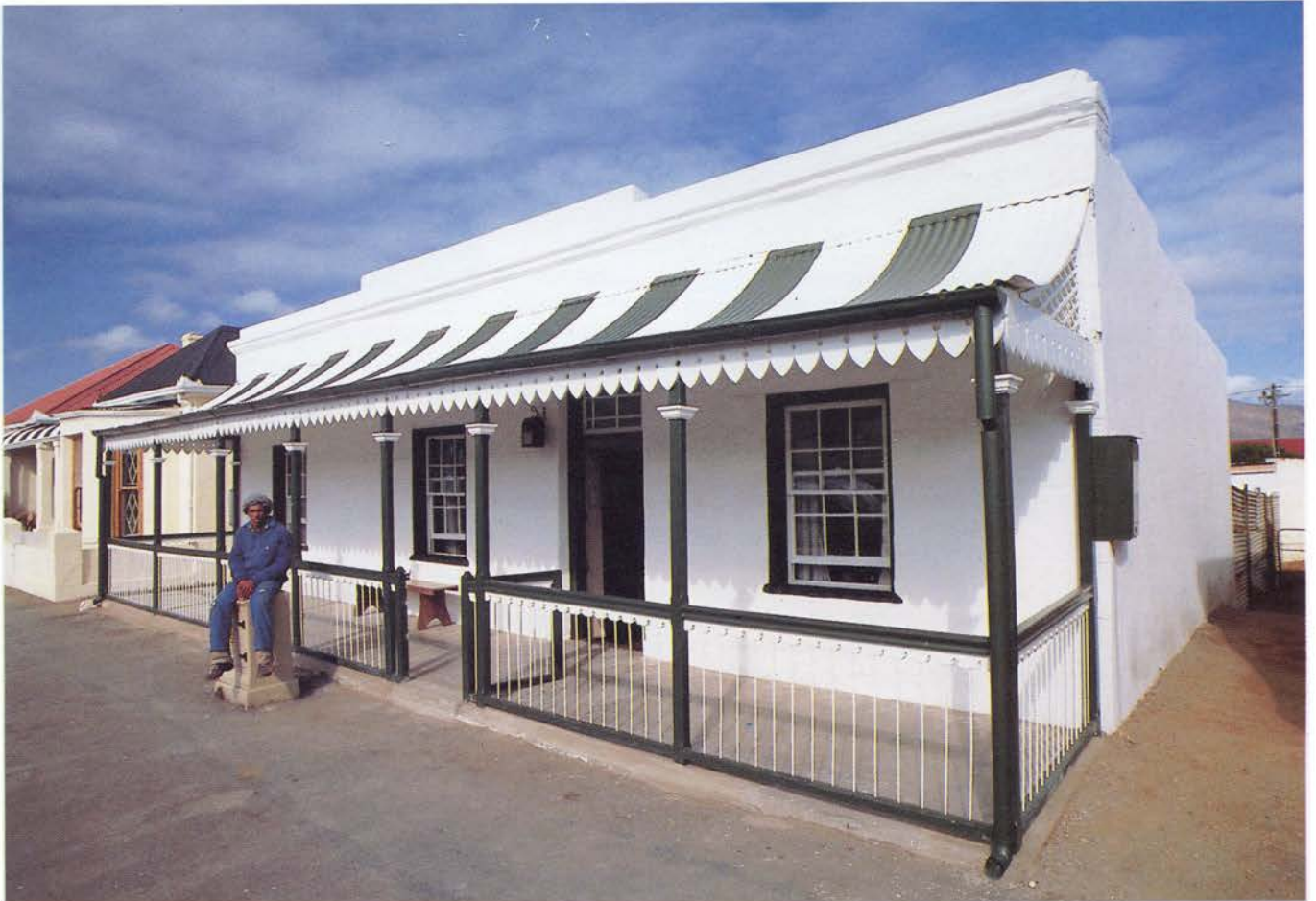
Above: An example of the renovated cottages in Market Street, Cradock
