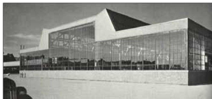
Figure 4 Dodge truck assembly plant in Detroit (Michigan) designed by Albert Kahn and constructed in 1937. The roof structure makes provision for additional light in the central portion of the building (source: Foster 1982: 116).
