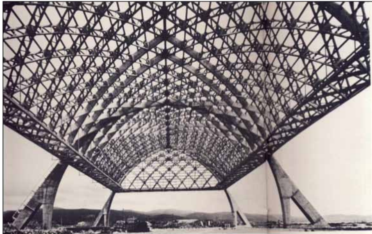
Figure 6 Completed structure of an airplane hangar at Orbetello (Italy) in 1939 constructed with pre-cast reinforced concrete. Designed by Pier Luigi Nervi, destroyed during the Second World War (source: Foster 1982: 143).
