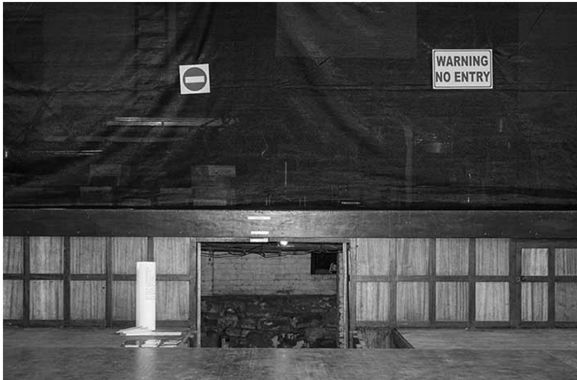
Figure 6 View of under-stage storage space entrance from main hall, Potchefstroom City Hall, 2012 (photo: courtesy of artists).
