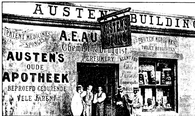
Fig. 8. Austen's Building, Cradock.
