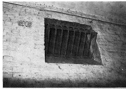
Barred cell window in the older part of Roeland Street Prison.
