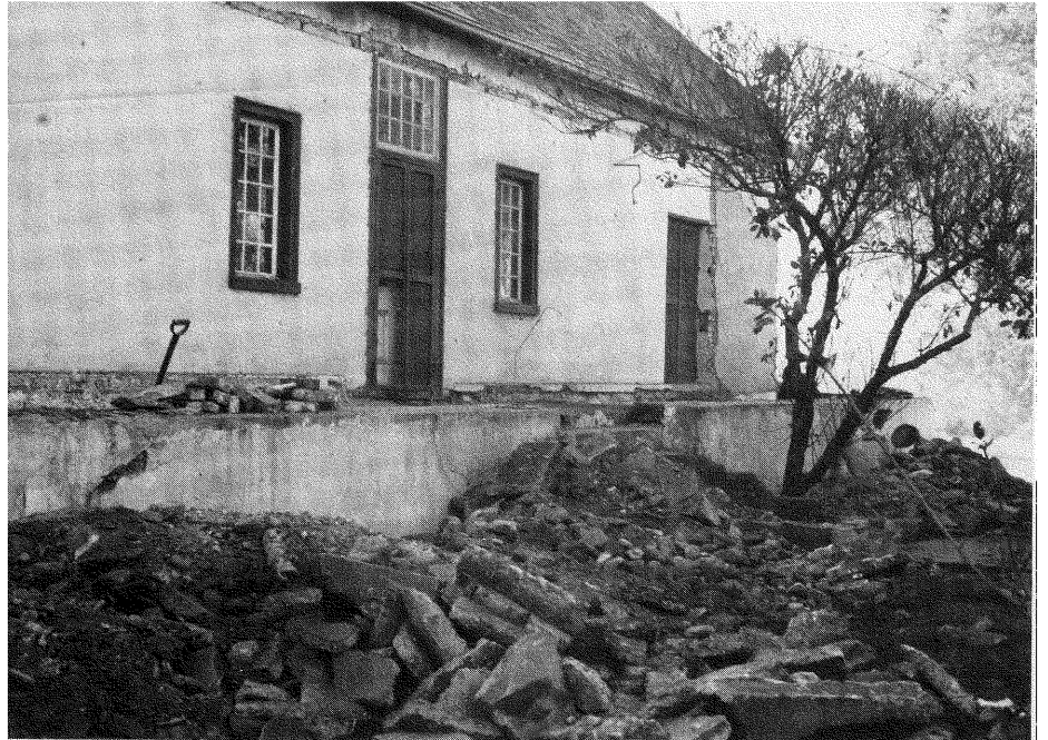
Cuyler Manor, June 1975, during removal of verandahs.
