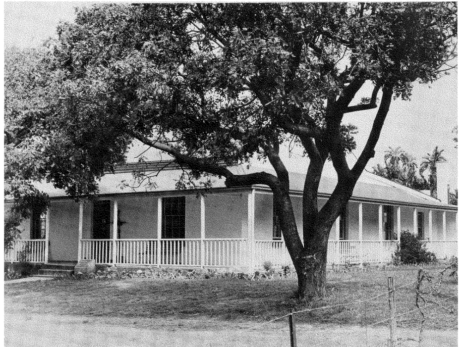
Gately House, East London – facade and west side.
