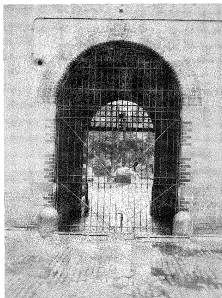
Main entrance as seen from the courtyard.
