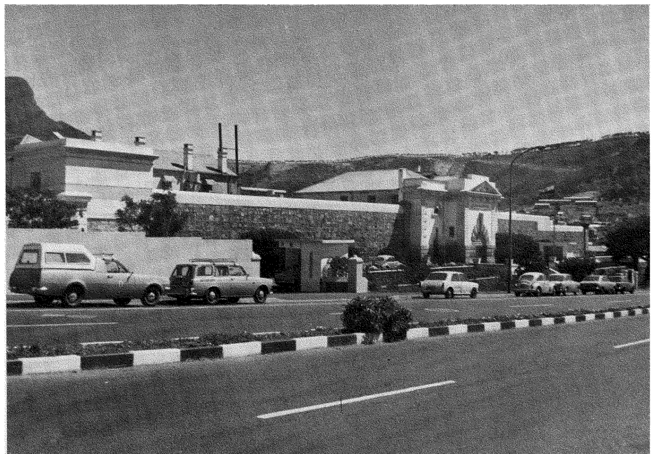
Roeland Street Prison, Cape Town—front view.
