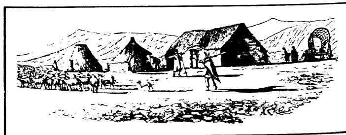
Fig. 2: Veldt Cornet Snyman's house in the Roggeveld, c.1810. From Burchell's Travels .
