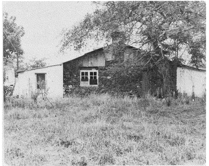
8. West view of the unrestored house in 1975. The later additions (white-washed brick) can be readily distinguished from the original stonework.
