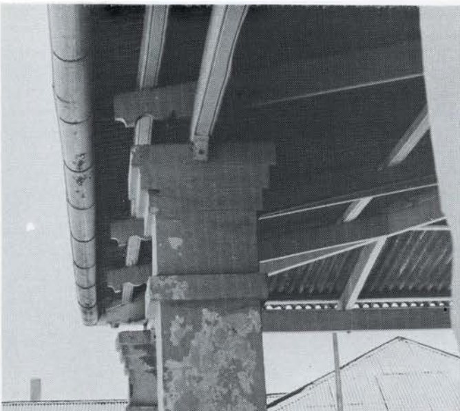
Fig. 25 Directorate of Building Services, Veranda details in the additions to the house of the Deputy Troop Commander, Windhoek, 1902. (Photograph 1979)
