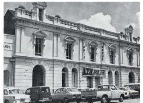
India House, Victoria Street, Salisbury.
