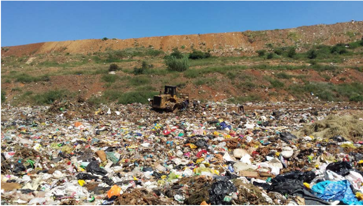
Figure 10: Processing of waste at the landfill site
