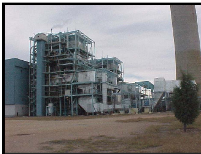
Figure 1. Thermoelectric Power Plant "Villa de Reyes"
