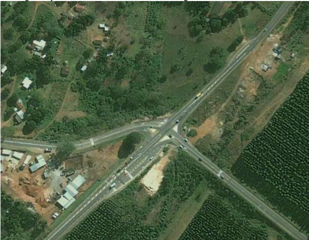
Figure2: R102 / P535 intersection before upgrades
