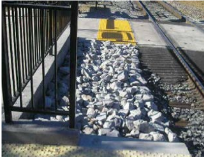
Figure 11(j): Track ballast discouraging pedestrian movement. Clark (2008)
