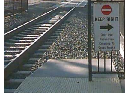
Figure 11(l): The length of ballast helps discourage pedestrians from using this route. Clark (2008)
