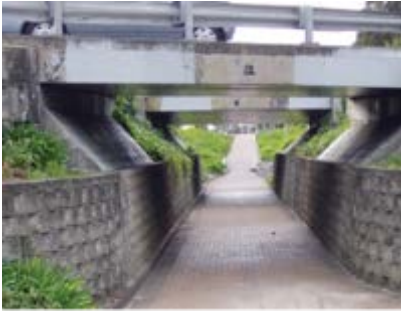
Figure 11(g): Pedestrian underpass. Clark (2008)
