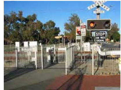
Figure 11(c): Lockable Gates, (web. FHWA, 2007)
