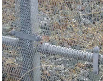
Figure 11(k): Close up view of security fencing. Clark (2008)
