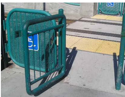
Figure 11(d): Warning Tactile ground surface Indicators, (Clark, May 2008)
