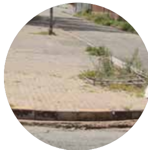
asphalt and paving
