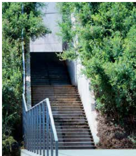
Figure 3.20. (left) Buried landing of the observation deck
