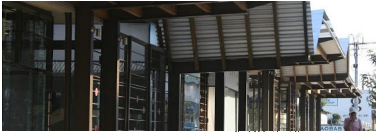
Fig. 3.32:Parkhurst Shops canopy
