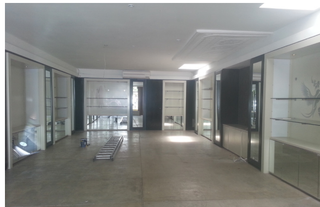
Fig. 3.35: Parkhurst store interior fit out
