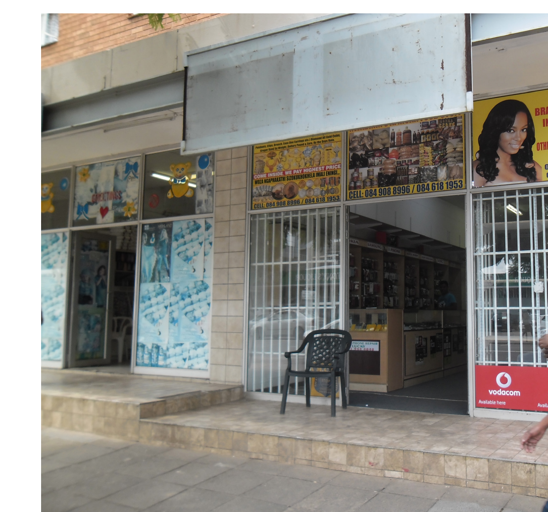
Fig. 4.43: Missing and incorrect signage
