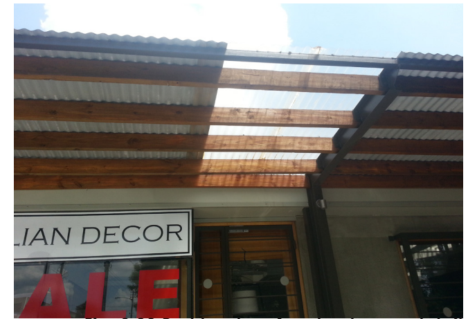
Fig. 3.39: Parkhurst roof and entrance detail
