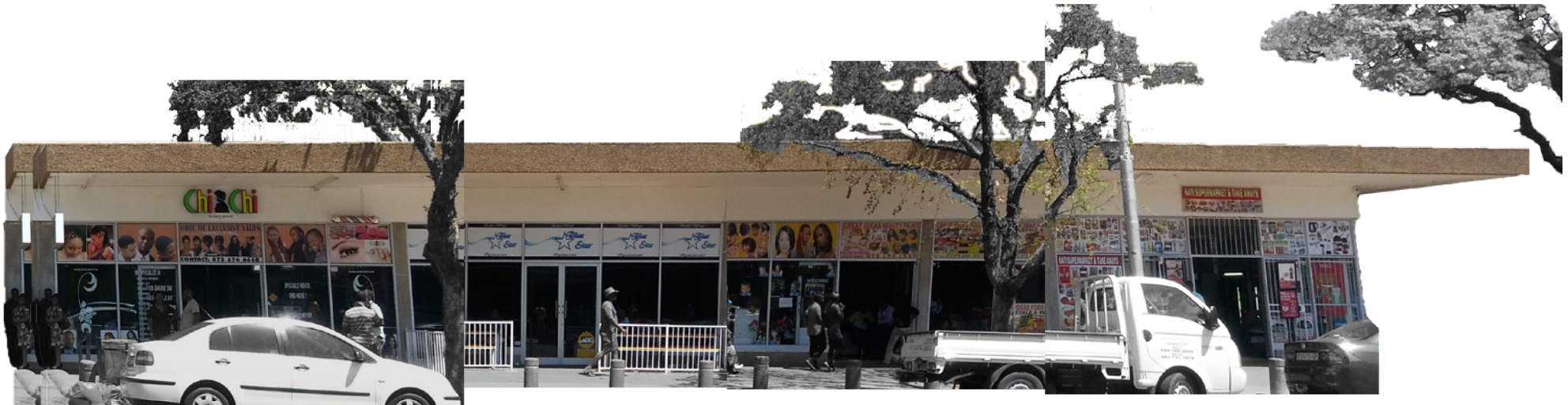
Fig. 4.24: Sunny Rock north facade
