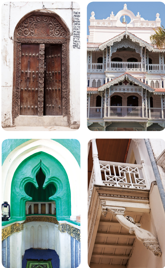
fig. 02.08_European, Arab and South Asian designs blended to form Zanzibar's distinctive architecture. Restored Old dispensary. 12th century mosque in Kizimkazi for Persian traders. Mosque door. Old dispensary balcony shows South asian influences.
