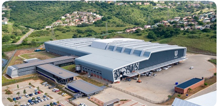
fig. 07.03 Aerial photo of the Unilever building, office block (left) and industry (right).
