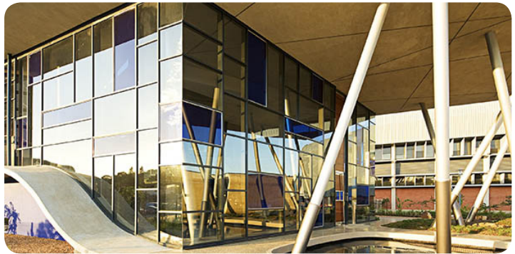
fig. 07.02 Perspective of glass and structural work at the offices
