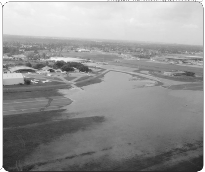
fig. 04.21_Zanzibar Airport flooded in May 2002.
