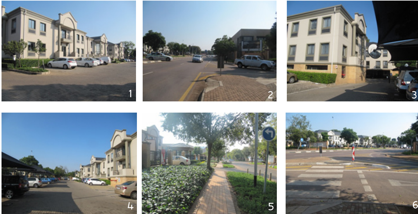
Fig 3.24: Site photos (by author, September 2014)
