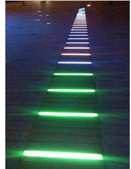
Fig 8.7: Permeable pavers with illuminating paving stones at 1200mm intervals ( www.smartstones.co.za )
