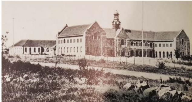
Fig 3.6: Photo of the Old Arts building directly after construction in 1910 (Tukkie Blad, 1970)
