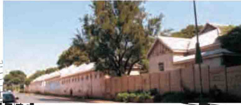
Railway compound (declare provincial heritage site)
