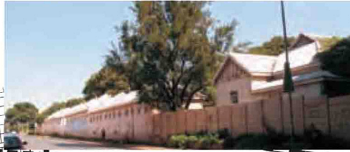
Railway compound (declare provincial heritage site)
