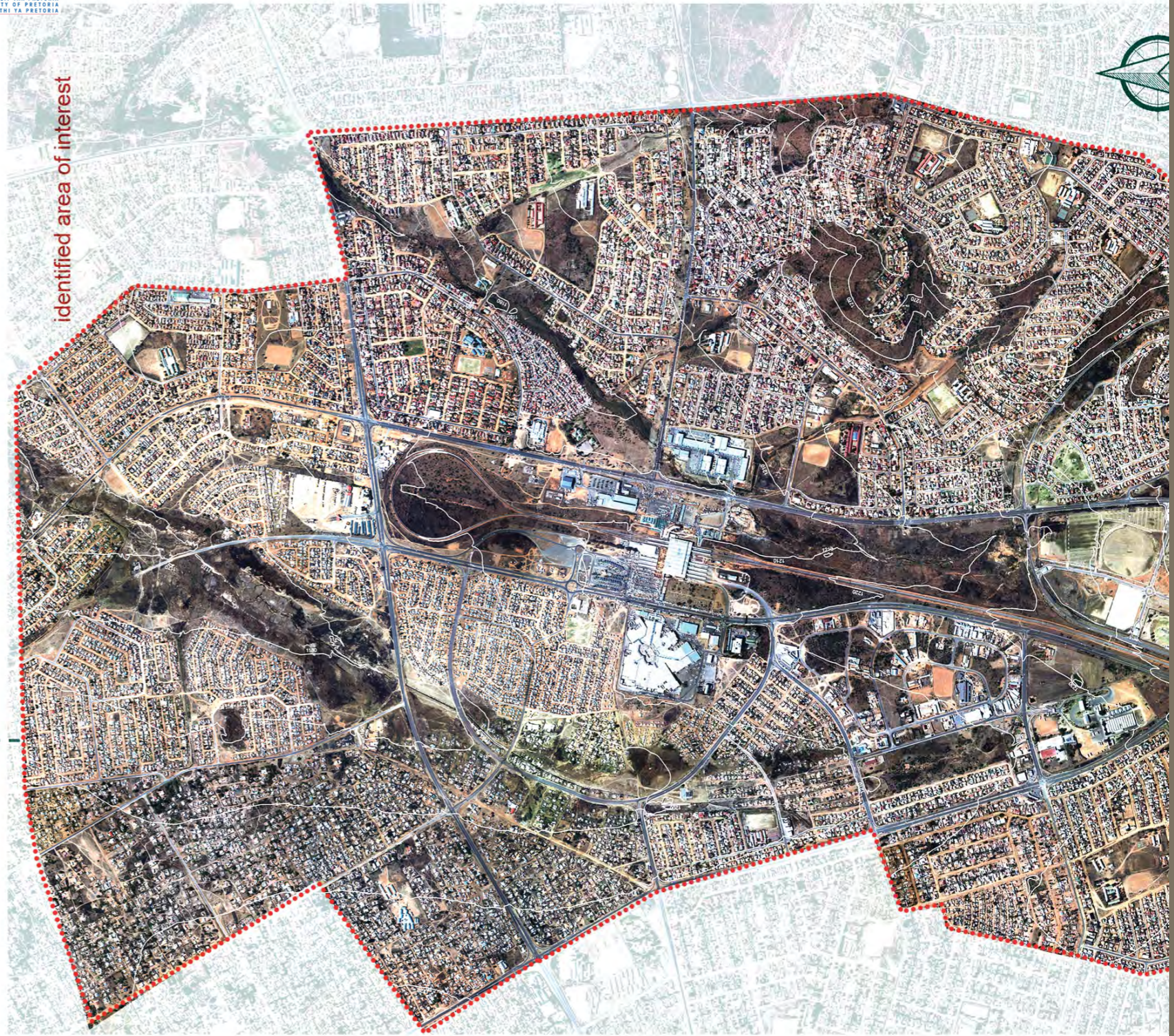
Fig 02-3 locality and infrastructure (Author, 2014)
