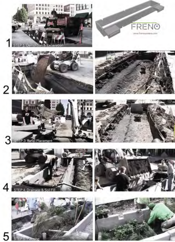
Fig 09-4g The raingarden system assembly and process (Freno systems 2014)
