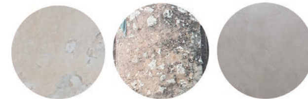
Figure 8.5 Recycled aggregate lime concrete with sliding formwork and lime/cement plaster render
