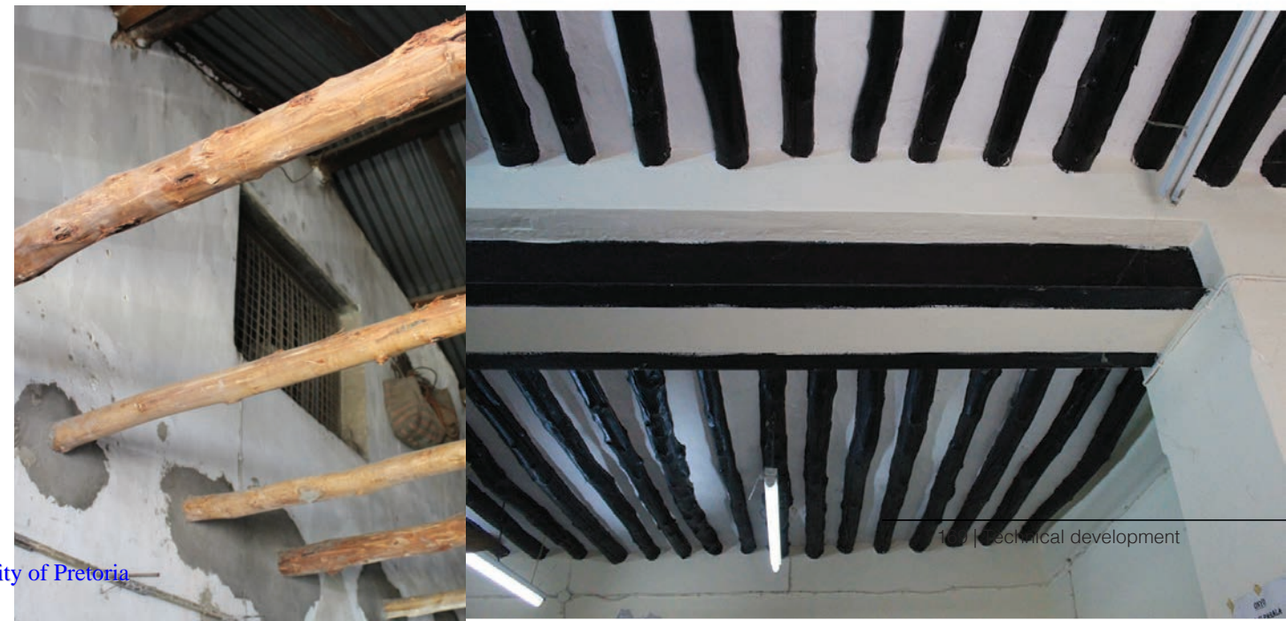
Figure 8.10 Traditional floor construction with mangrove poles
