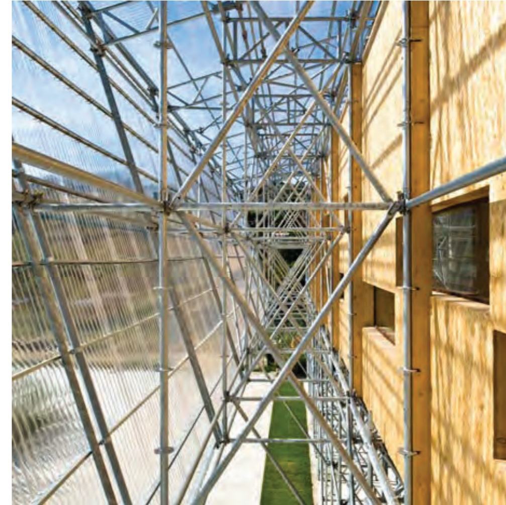
Figure 4.60. EXISTING BUILDING STRUCTURE (SANCEREAU 2011)
