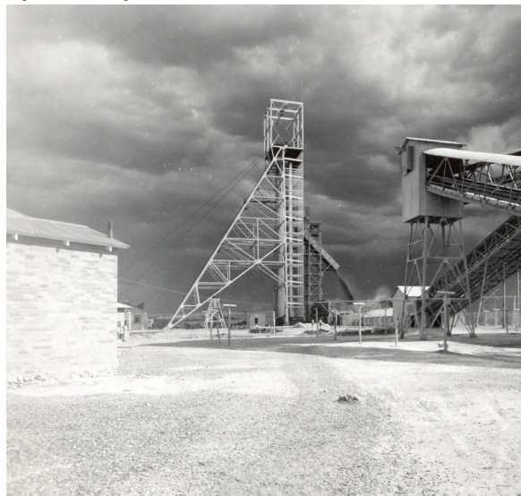
Figure 3.6. Mine structures (Cullinan archives, 2014)
