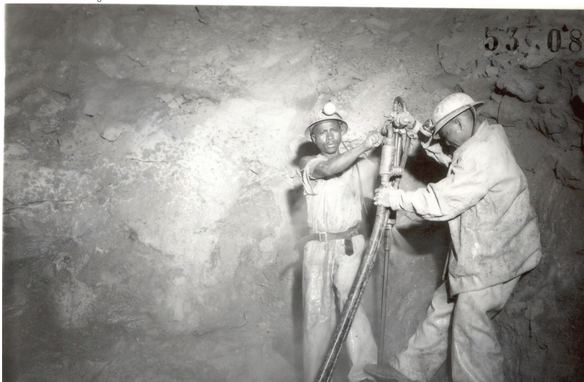
Figure 3.4. Subsurface drilling (Cullinan archives, 2014)
