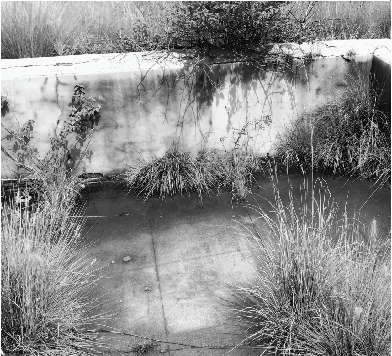
Figure 3.21. Concrete bath, emptied (2014)
